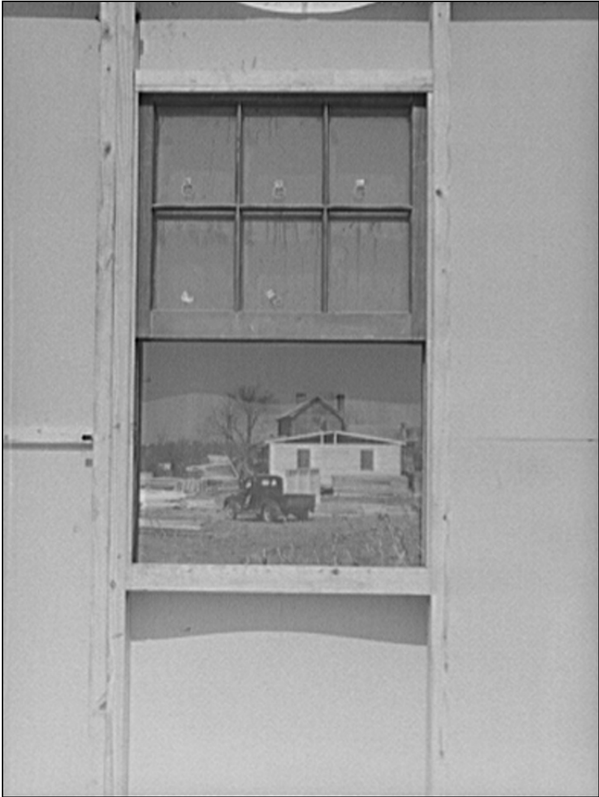
Picture Caption: Prefabricated houses being built to house some of the farmers who had to move out of the Camp Croft area. Pacolet, South Carolina
