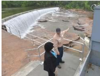
MICHAEL JUSTUS/michael.justus@shj.com Mike Callahan, of Lockhart Power, right, leads Damaron Anderson, of the S.C. Commission for the Blind, on a tour of the Pacolet hydroelectric plant Thursday morning during an open house at the facility.
