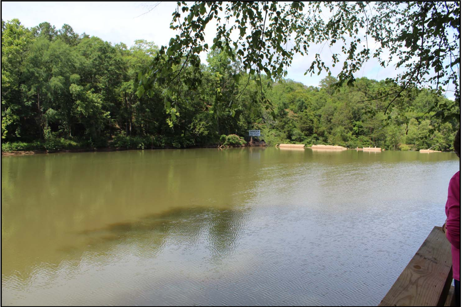
Looking downstream towards the dam .
