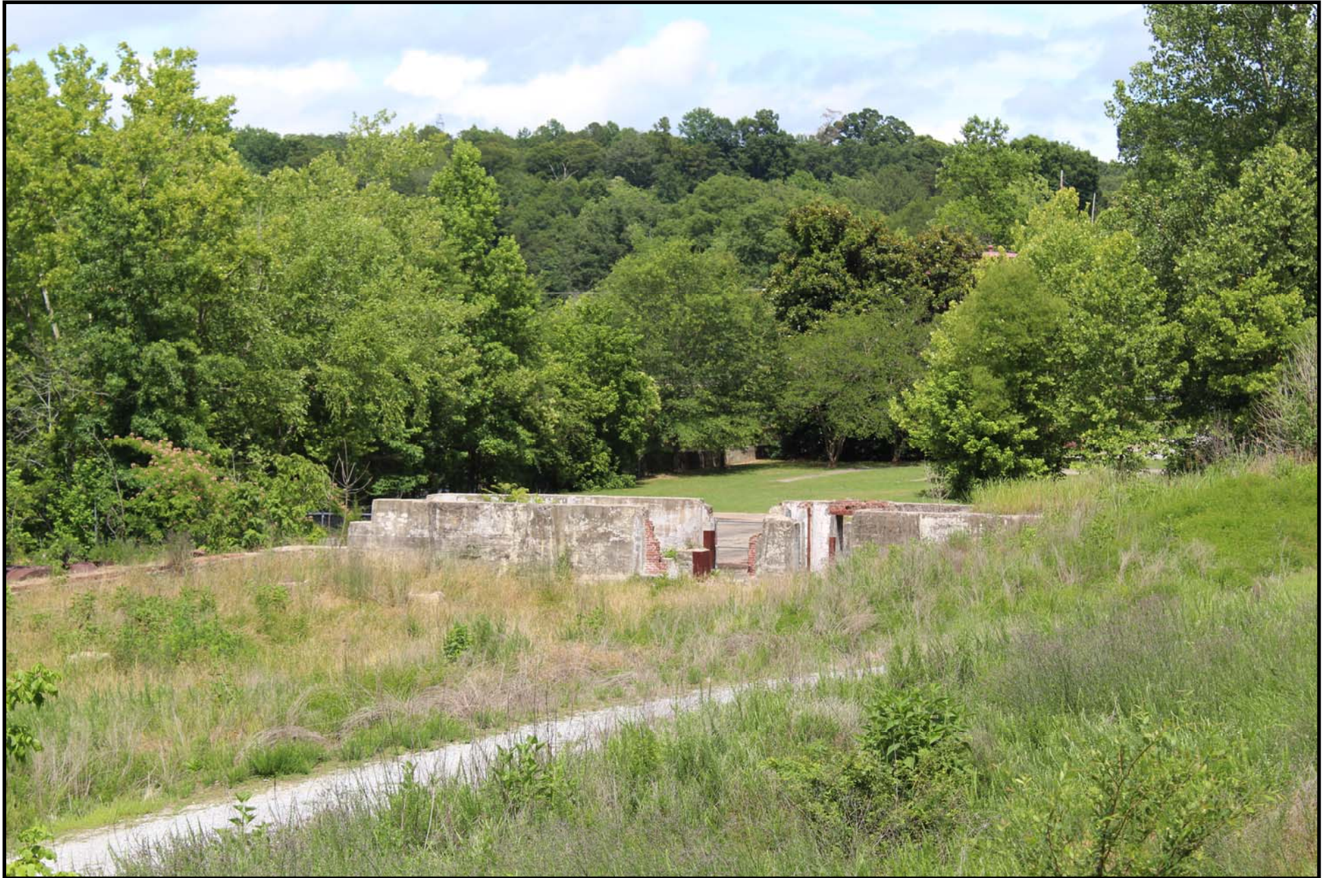
Part of the remaining foundation for the “New Mill” or Mill Number 5. Looking toward the Pacolet River which is beyond the line of trees.
