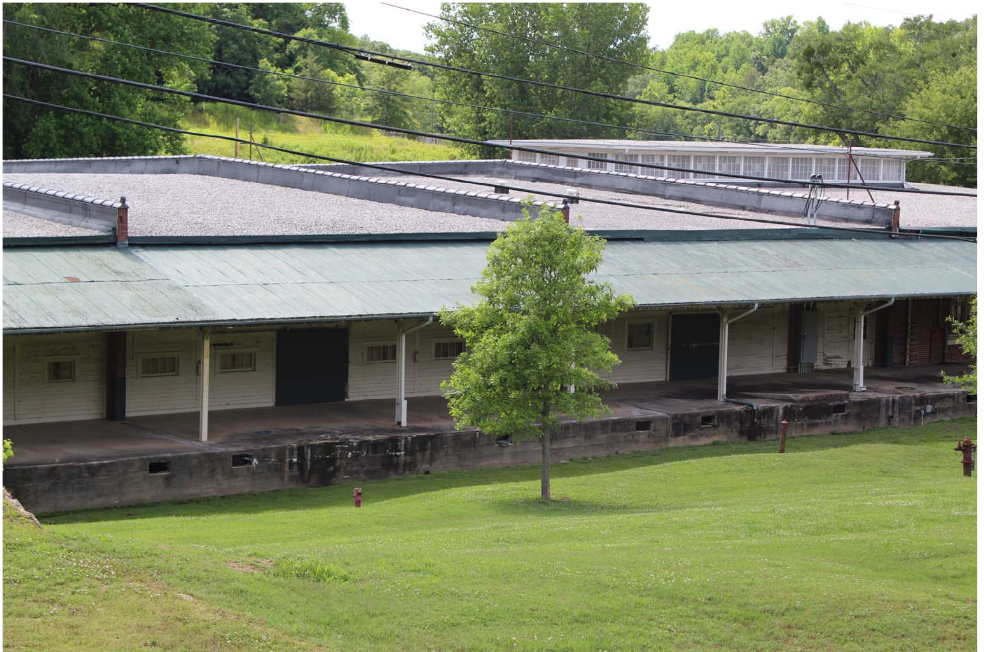
A closer view of the Cloth Room . When it was in operation, the railroad tracks for the Dummy ran right alongside the loading dock.
